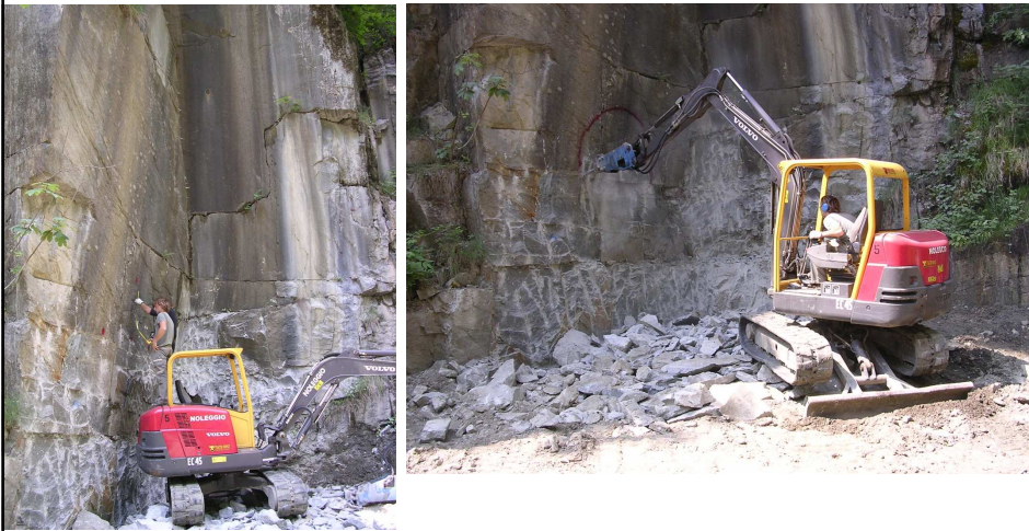
Construction of the test site
